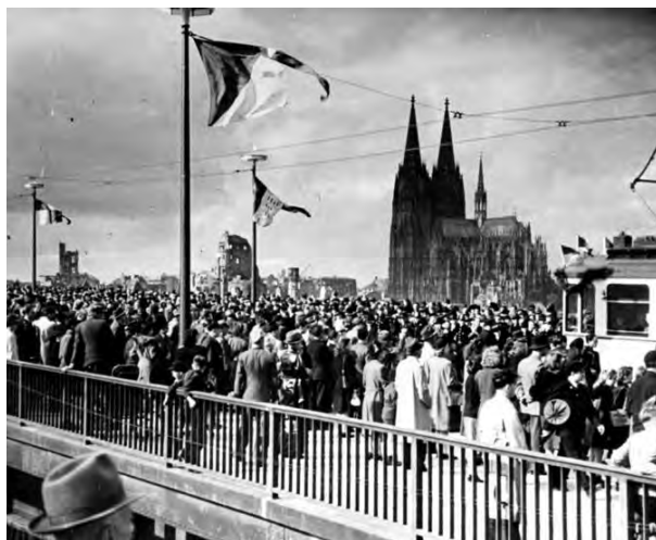
Inauguration of the Detz Bridge, first german bridge rebuilt after the war, 1948
