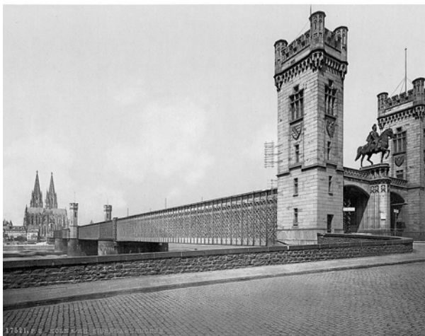
Cologne built his first railway bridge in 1855
