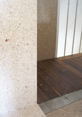
Conservation of the existing floor, concrete reprise of the chute, and the set of multi-function panels (MFP) on the floor and walls of the refurbished room Bagnole, France (93)
