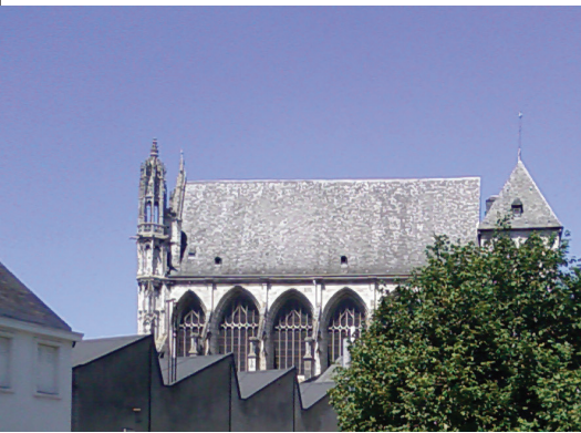
View of the collegiate church and factory behind the property of the Nauzes Vernon, France (27)
