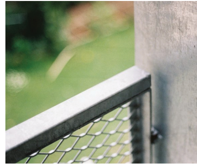
Detail of the galvanized steel handrail Vernon, France (27)
