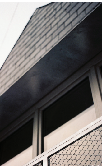
Above, view of the garage structure below the Studiolo. The existing walls were left as-is. The materials for the extension were chosen for their low cost and "raw" materiality.
