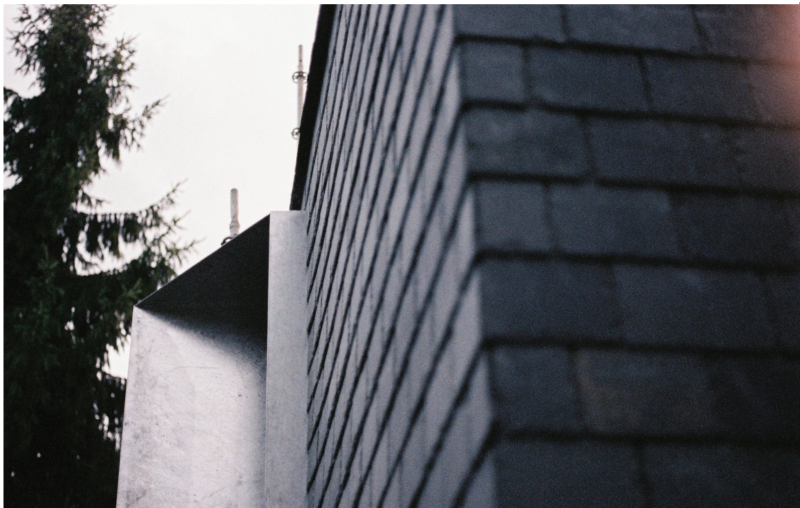
View of the light catching of the galvanized steel and the slated siding Vernon, France (27)
