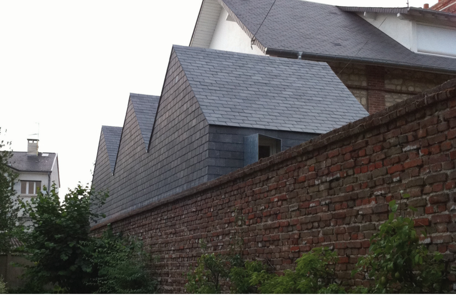
View from the street of the built extension Vernon, France (27)
